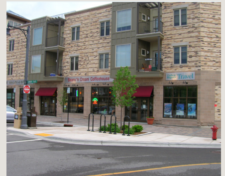
First floor retail with upper story office or residential with shallow setbacks.
