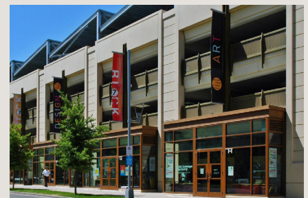
Design for a parking structure along a public street should provide visual interest compatible with adjacent developments and is encouraged to provide occupiable spaces along the street level.
