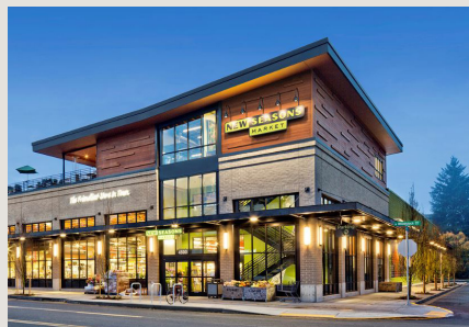
Two stories (or the appearance of two stories) should be the minimum building height in the DMU area. Development should hold street corners by extending the building facade (and roofline) higher at least one bay deep from the corner.
