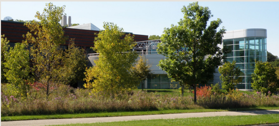
Using generous amounts of landscaping to screen large industrial buildings from street view.
