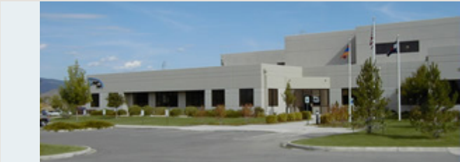
Variations in facade depth and heights for industrial buildings to break up long monotonous walls.
