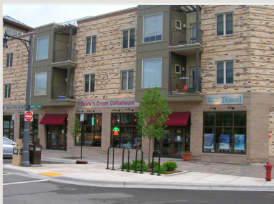
First floor retail with upper story office or residences is preferred with shallow setbacks to promote walkability.
