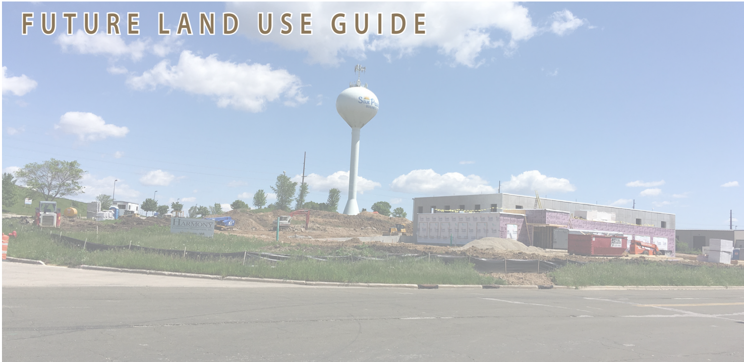
Construction of MacDon Enterprises' New Facility in Business Park
