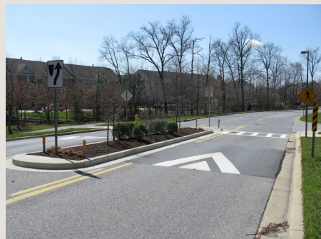
Raised Median / Crossing Refuge, Plus Speed Table
