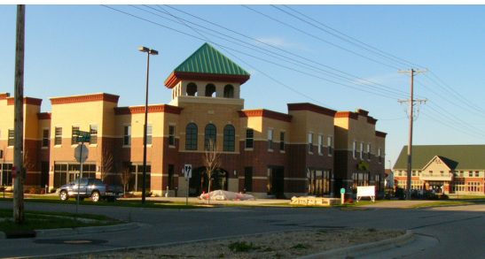
Commercial Node (Liberty Blvd)
