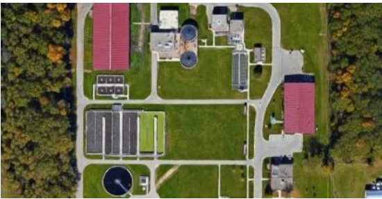
City Wastewater Treatment Plant
