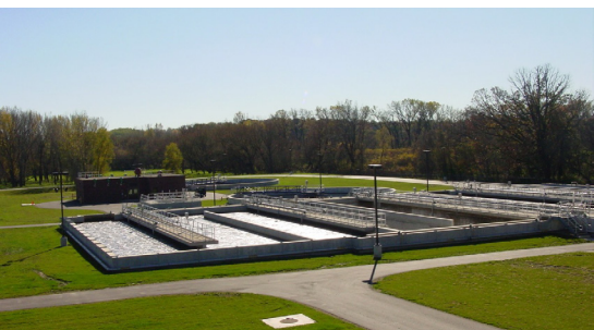
Activated Sludge Basins
