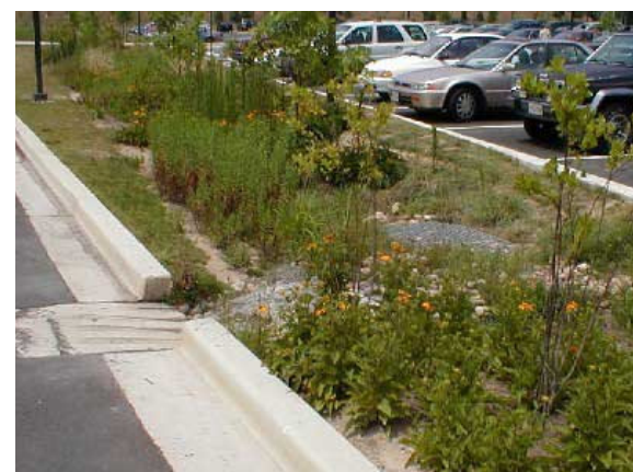
Rain Garden in Commercial Parking Lot
