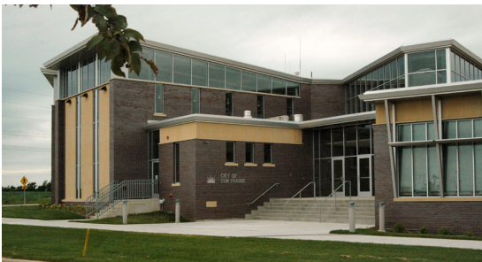
Westside Community Service Building
