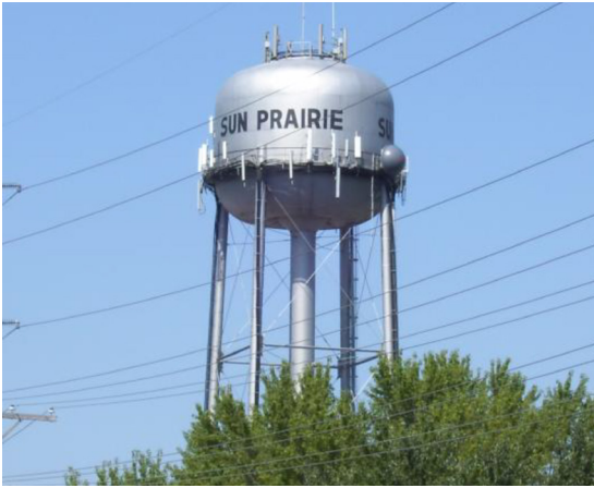
N. Bird Street Water Tower
