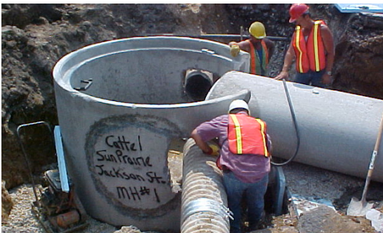
W. Main Street Sewer Installation
