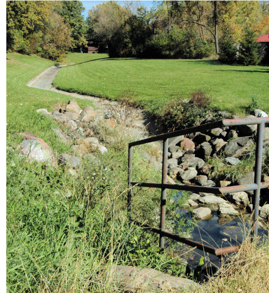
Example of Stormwater Management
