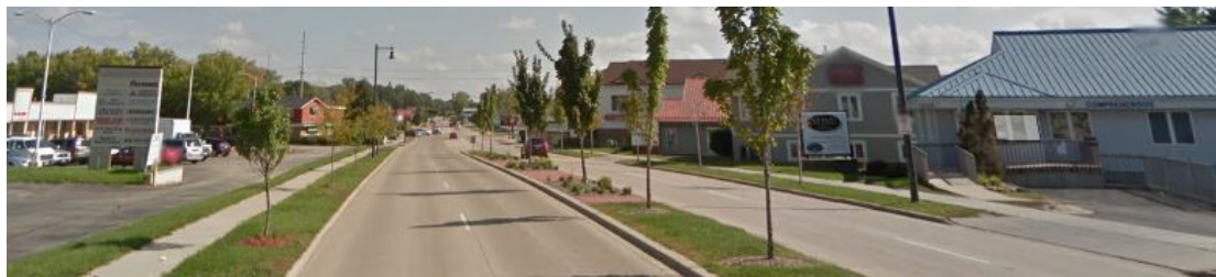
TOP Example of dated architecture in the corridor MIDDLE Example of new construction LEFT W. Main Street Section
