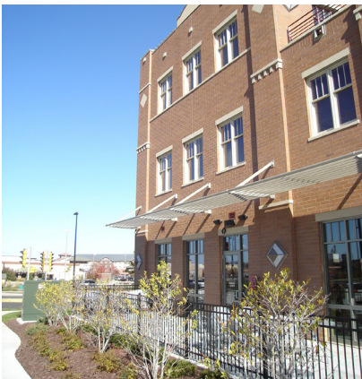
LEFT and BELOW Example of medium-density mixed-use development with ground floor retail
