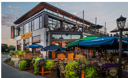
LEFT Design standards showcasing an attractive façade, building materials, and site layout
