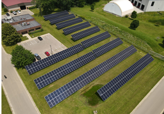
Solar Installation at City Wastewater Treatment Plant
