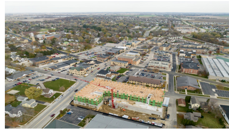
The Monarch Redevelopment, 110 S .Bristol St.
