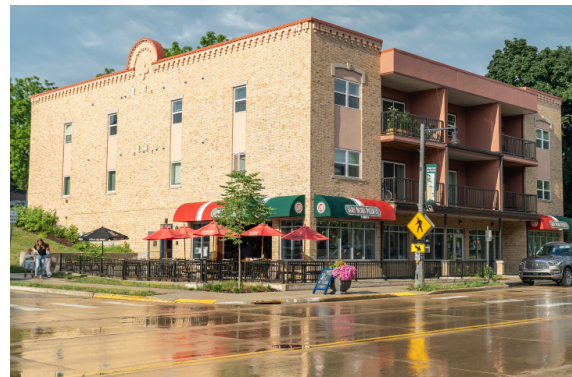
TID 14 - Bougie Building, 410 E. Main St.
