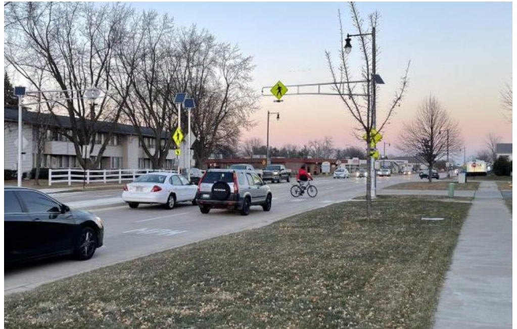
Figure 2: Sun Prairie recently installed an RRFB at W Main Street and Hart Road as part of Vision Zero efforts to improve safety along the corridor
