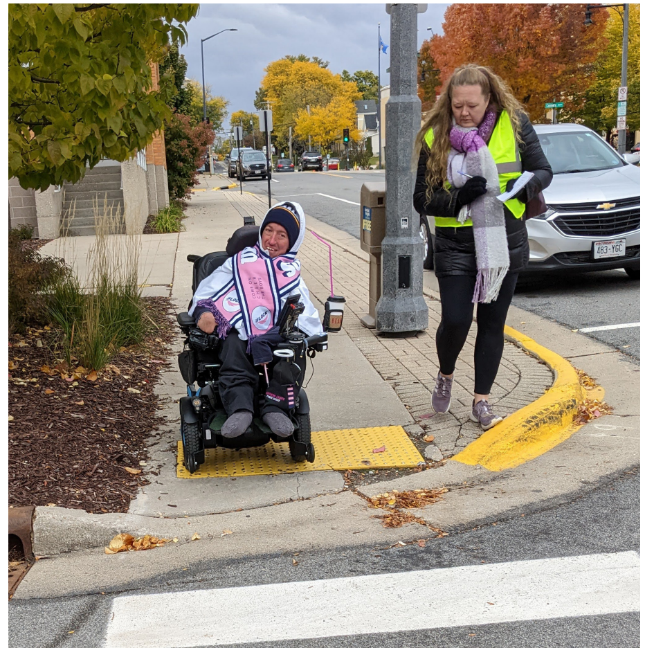
The Fall 2022 group walk demonstrated many accessibility concerns in downtown Sun Prairie, including this curb ramp which is missing pavement and could have tipped this participant’s mobility scooter if the front wheel had gotten caught.
