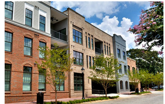
Concealed Parking Deck
